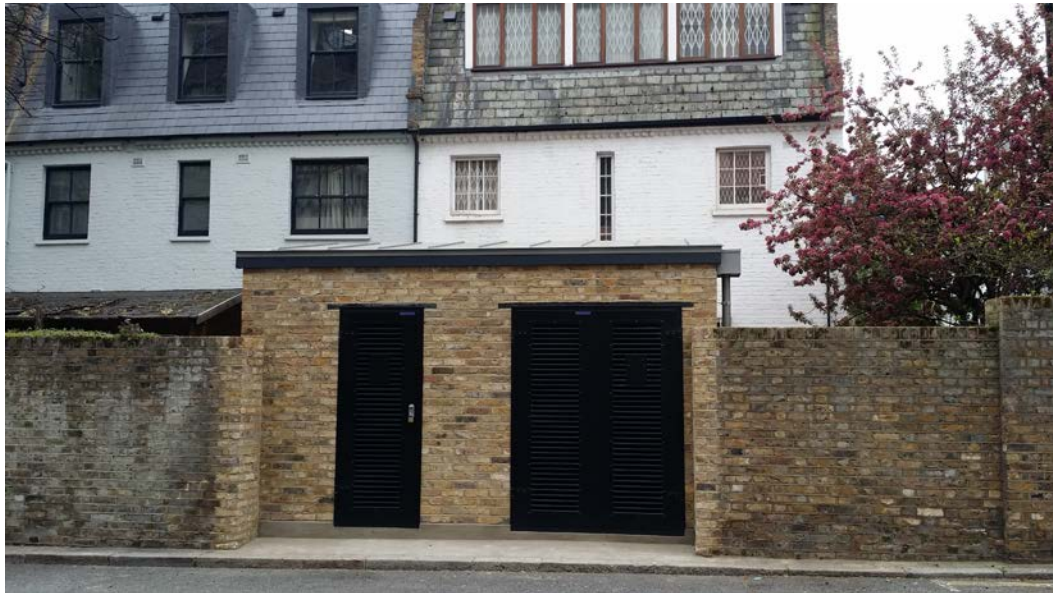
Photo to shows doors
